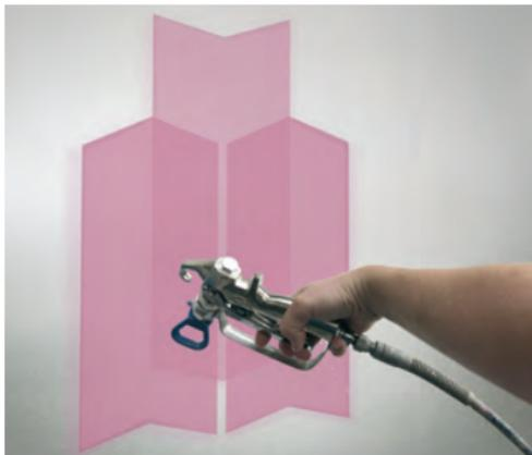
**18 inches** from the surface and spray horizontal passes followed by a vertical passes working slowly over the surface in manageable sections.
